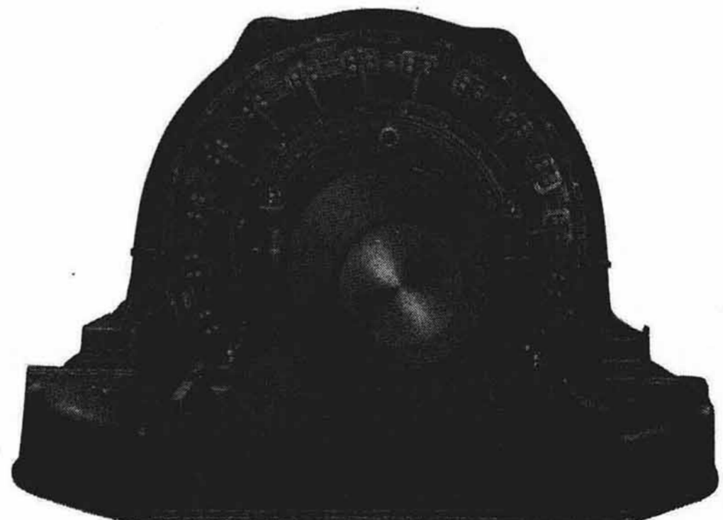
Side View of 23,600 HP Double Armature Type Reversing D.C. Motor
