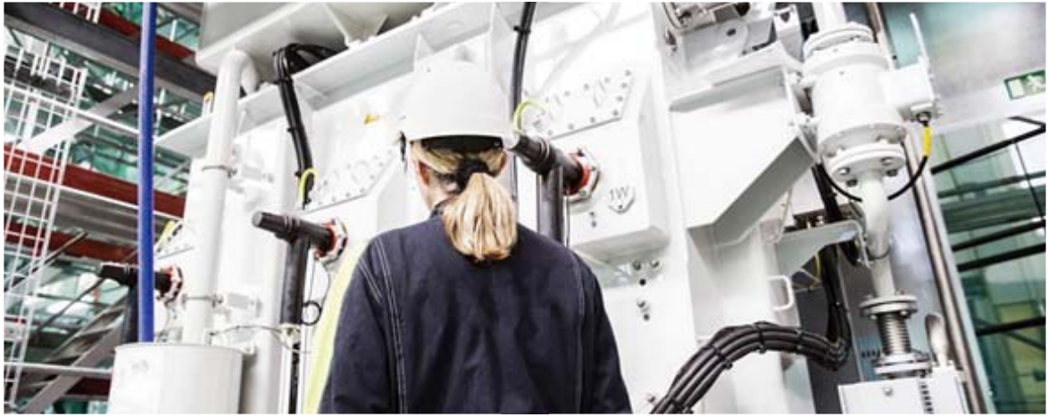
29 66 kV変圧器WindSTAR
