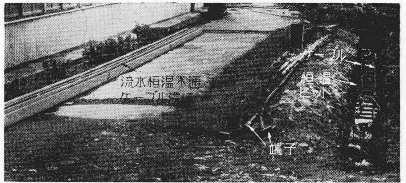
第6図 試料の温度調節装置外観 Fig.6. Outside View of the Temperature Control Installation
