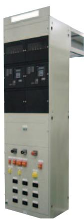
**12** Digital protection relay equipment for phase modifiers
