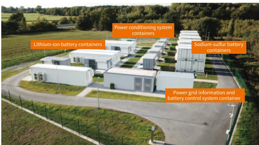
7 Large-scale hybrid power storage system demonstrating operation (photo courtesy of NEDO and EWE AG)
