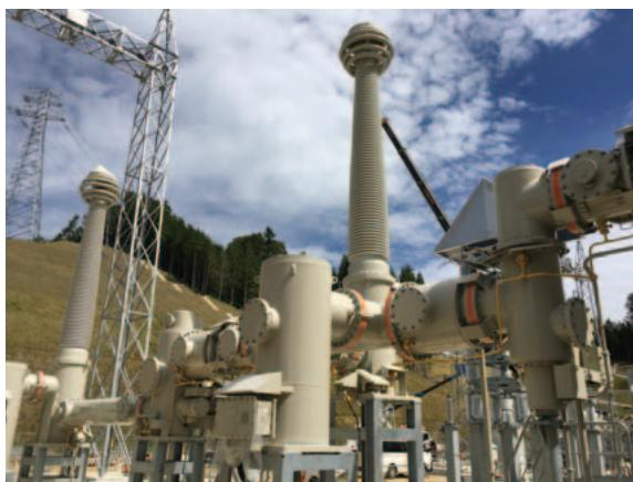
8 DC gas-insulated switchgear (DC200 kV)
