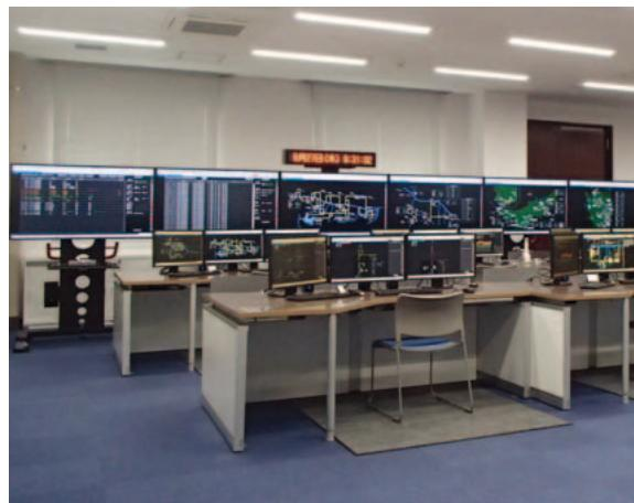
3 Large screen display and monitoring/control panels for Tohoku EPCO's Hydropower Operation Center Southern System
