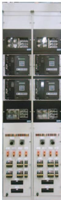
1 Transmission line protective relay device
