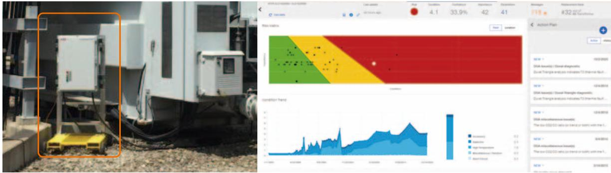
33 Remote monitoring using mobile CoreSense™ M10 (left) and diagnostic APM dashboard showing real time transformer condition
