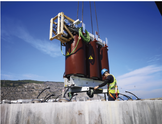
[05] Erection of the CompactCool unit inside the tower of Saitec
