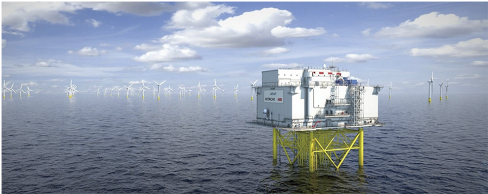
[06] An offshore converter station at Dogger Bank, United Kingdom (Source: Hitachi Energy; Credit: Aibel)
