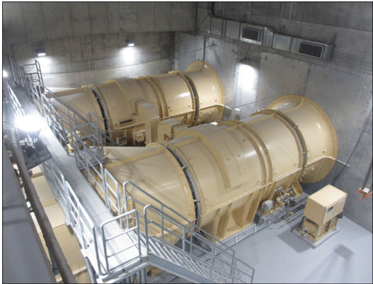
[03] Two Exhaust Fans (Variable Blade Axial Flow Fan) Installed at Tsukiji Ventilation Station
