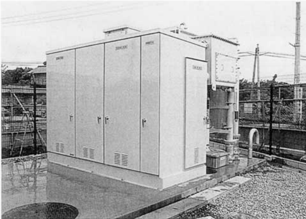
Fig. 9— External View of Distribution Tower. Switchgear with multi-functional vacuum interrupters is shown in the foreground in front of the 10-MVA transformer. External dimensions are 3.65 m (W) \times 4.1 m (D) with an installation area of 15 m 2 .
