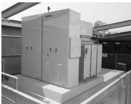
(a) External view of power-distribution facilities using switchgear with multi-functional vacuum interrupter
