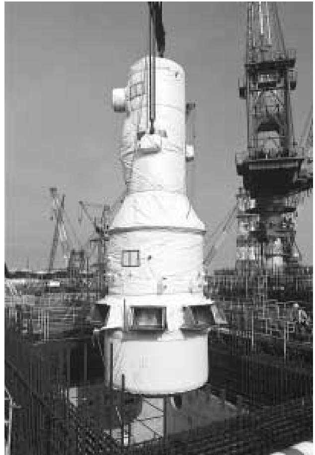
Fig. 3— Installation of Apparatus for the Concentration of High-Level Liquid Waste; Corrosion-Resistance Techniques Were Gathered on a Worldwide Scale for Application to This Waste-Reduction Vessel.
