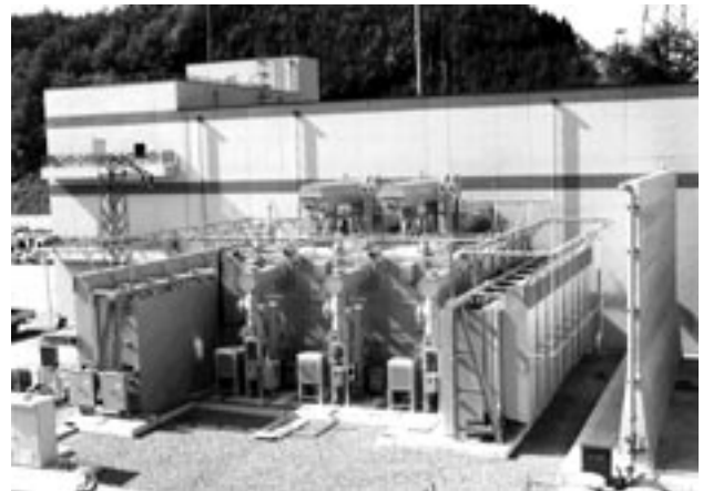
Fig. 7— 872-MVA Converter Transformer (Kihoku Converter Station).
