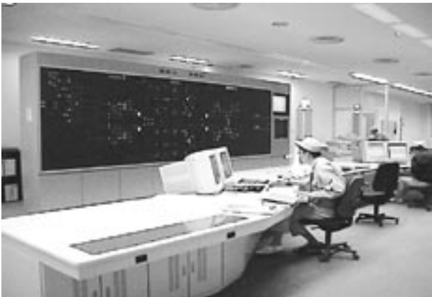
Fig. 9— Substation Control System of the Kihoku Converter Station.
