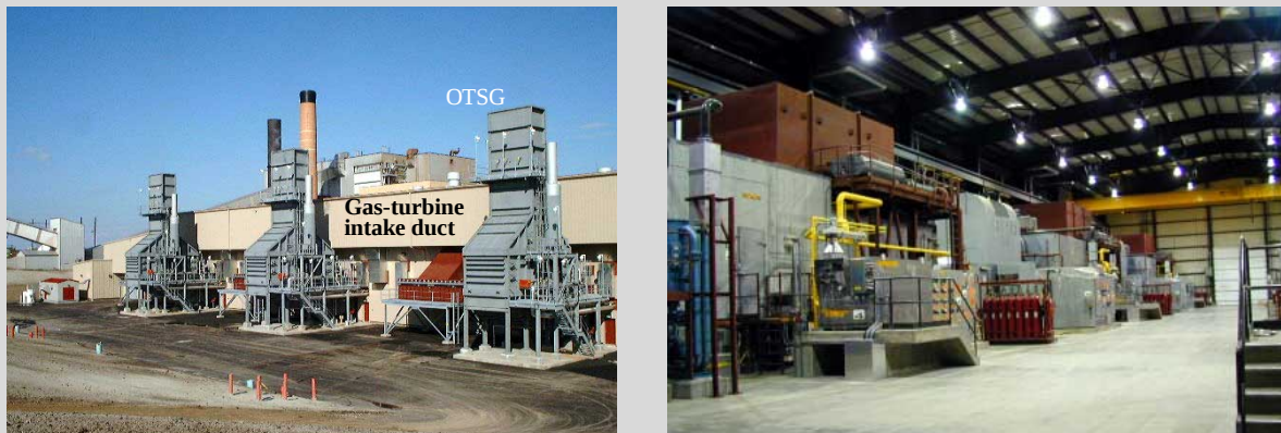
Fig. 1—Re-powering System Installed at Queen Elizabeth Power Station (on the left); H-25 Gas-turbine Units (right).
