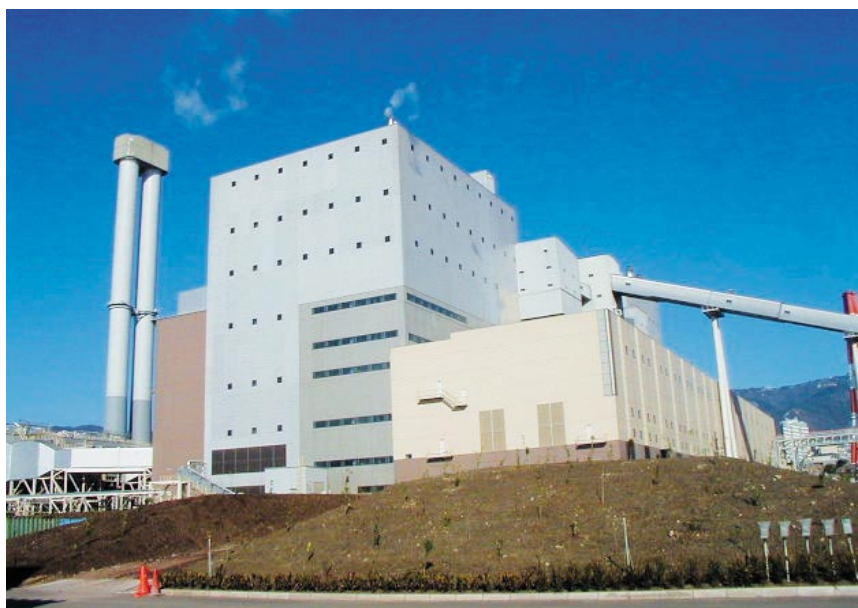
Fig. 1—Panoramic View of Shinko Kobe No.2 700-MW Power Station of Kobe Steel, Ltd.
