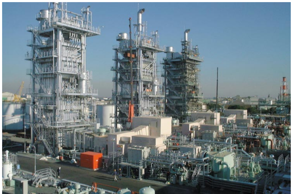
Fig. 1—External View of the Goi Power Plant of Goi Coast Energy, Ltd. Hitachi has completed three units of a single-shaft type combined-cycle power-generation plant on the premises of Chisso Petrochemical Corporation. Each plant consists of a gas turbine, generator, steam turbine, and heat recovery steam generator in a compact configuration.
