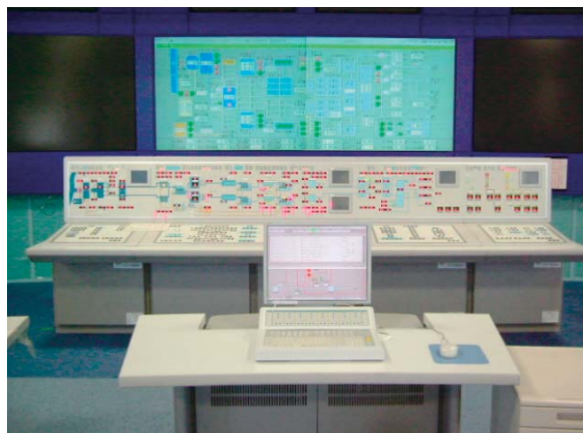
Central monitoring and control system at Niwakubo Water Treatment Plant, Osaka Waterworks Department
