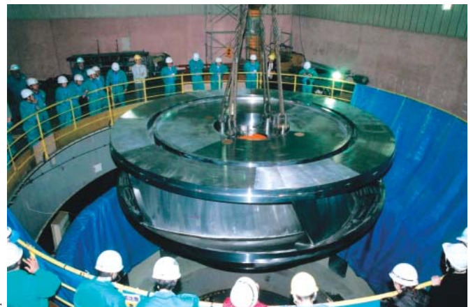
Installation of water-turbine runner
