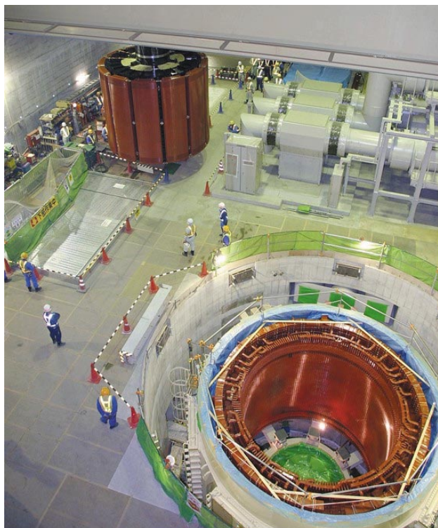
Fig. 3—Generator-motor Stator and Rotor.
