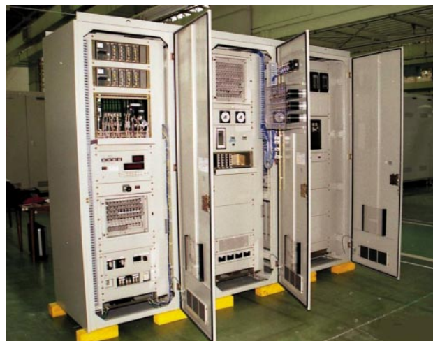
Fig. 7—Thyristor Starter Control and Protection System. Five panels have been reduced to three through reduction of hardware circuitry.
