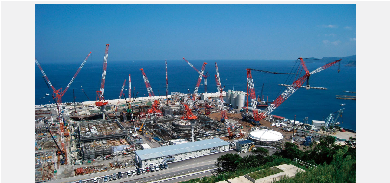
Fig. 1— Construction of Unit No. 3 at the Shimane Nuclear Power Station of The Chugoku Electric Power Co., Inc. The plant is being constructed using the latest construction methods including the large crawler crane at the right of the photograph. Equipment installation is now in progress with building and equipment construction proceeding in parallel.
