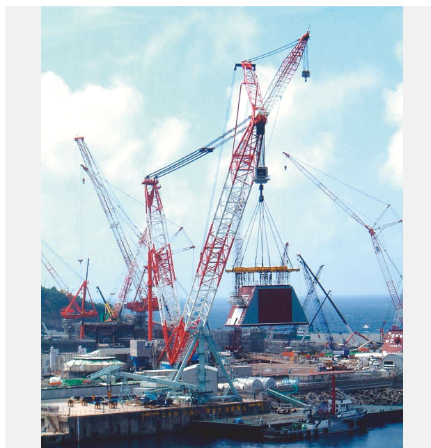
Fig. 4—Direct Unloading by Large Crawler Crane.
