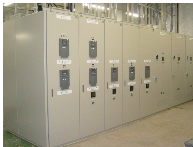
Fig. 7—View of Switchgear with Solid-insulated Bus Bars. Switchgear are installed at a substation for the Shinkansen rail system.
