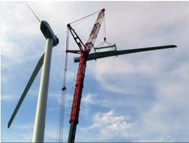
Fig. 6—Blade Being Attached to Hub at Top of Tower. Assembling the rotor in the air one blade at a time saves on ground space.
