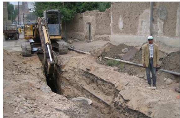
Fig. 5—Installation of Water Pipes in Yemen.
