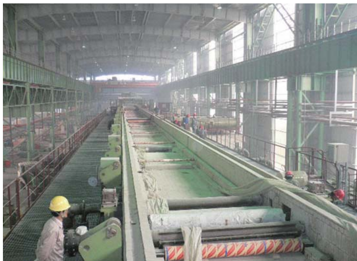
Pickling line during construction
