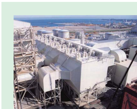
Moving electrode type electrostatic precipitator for coal fired power plant
