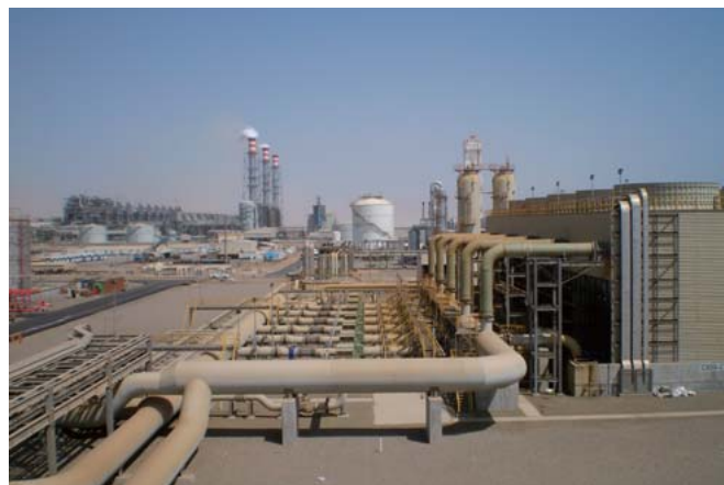
Cooling water supply system, part of the UO-1 utilities and off-site plant for Petro Rabigh in Saudi Arabia
