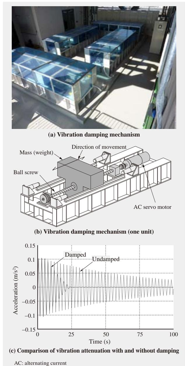
Fig. 7—Vibration Damping Mechanism. The vibration damping mechanism consists of four units, two each in the X and Y directions. The system damps vibrations by using an electric motor to move a weight.
