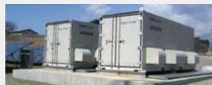
(b) PCS with FRT function to maintain operation during transient voltage drops
