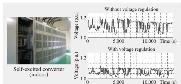
(a) Example of suppression of voltage fluctuation by STATCOM
