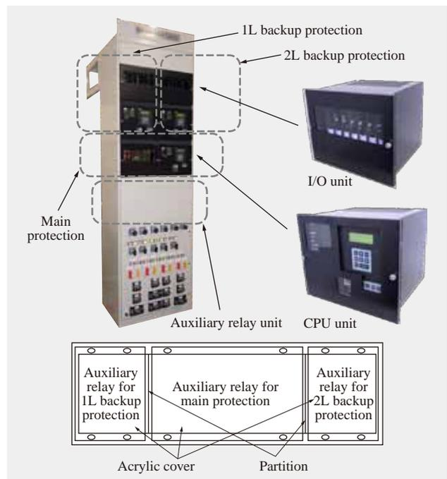
Fig. 6—Example Configuration for New Digital Relays. The system is configured by mounting the units that provide the functions and performance in a protection equipment panel. This allows functional modifications to be made by replacing units, with the swapping of components in and out being done on a unit-by-unit basis.
