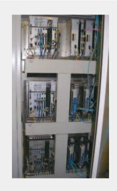
Fig. 3—Train Existence Supervision Equipment. The train existence supervision equipment tracks and supervises all of the trains controlled by the system, and provides backup functions in the event of a problem in the ground controllers.
