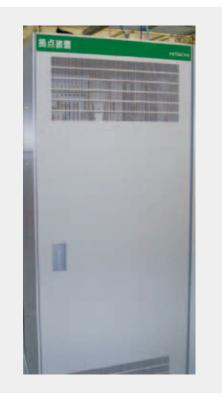
Fig. 2—Ground Controllers. The functions of the ground controllers include controlling the intervals between trains and calculating LMAs.
