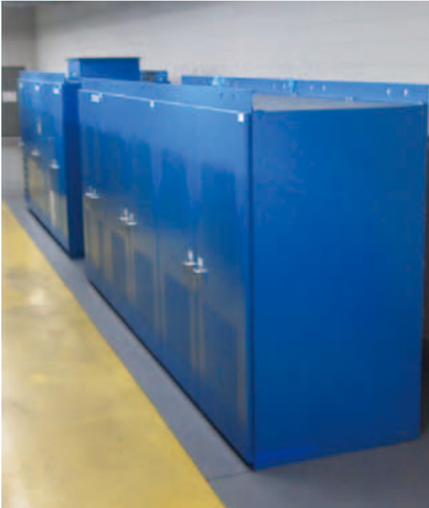
Fig. 9—System Storing Regenerative Electric Power in Wayside Storage Batteries on Seoul Metro9 Subway.
