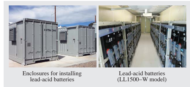
Fig. 7—Lead-acid Battery System Installed in Los Alamos County, New Mexico, USA.
