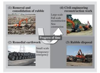
*Fig. 1—Progress over Time of Recovery and Reconstruction Work.*
