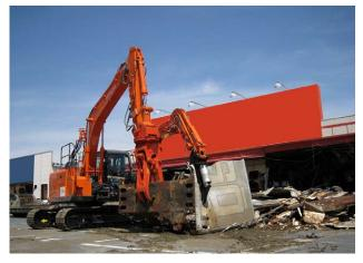
Fig. 4—Removal of Refrigerated Vehicle Containers (Ishinomaki City).
