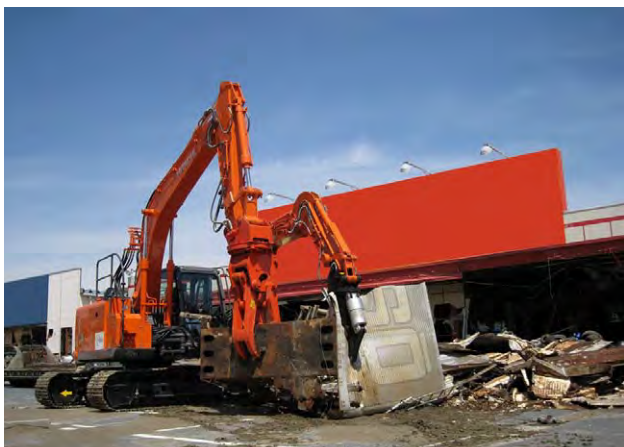
Fig. 4—Removal of Refrigerated Vehicle Containers (Ishinomaki City).
