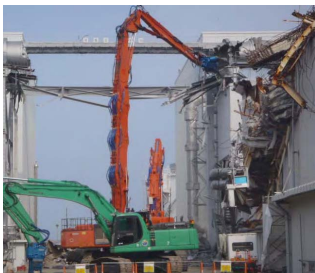
Fig. 8—Remotely Operated Upright Demolition Machine. Hitachi Construction Machinery's remotely operated demolition machine (center rear of photograph) in action at reactor No. 3 where it is used for tasks such as removing beams from the collapsed building.
