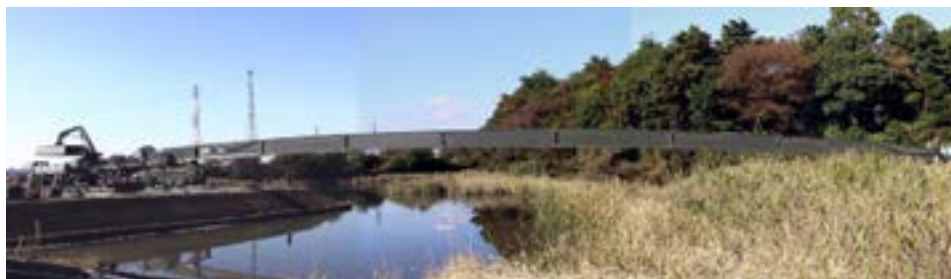
Fig. 4—Guide Beams during Deployment Process. The guide beams have a welded structure of high-strength aluminum.
