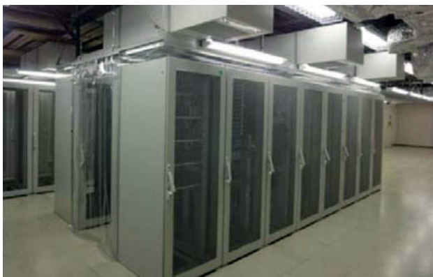
Fig. 4—Spot Cooling System Installation.
