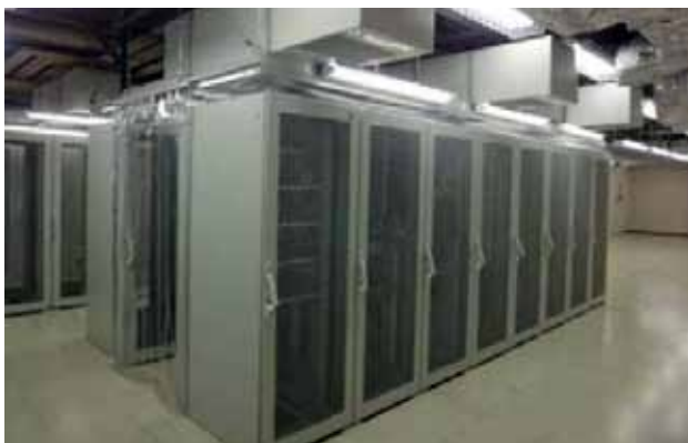
Fig. 4—Spot Cooling System Installation.
