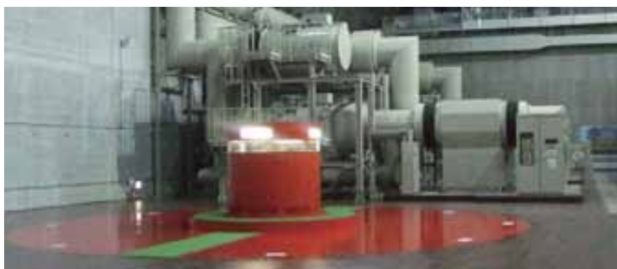
Unit 2 motor-generator at Kannagawa Hydroelectric Power Station of Tokyo Electric Power Co., Inc. (operating in pumped storage mode)
