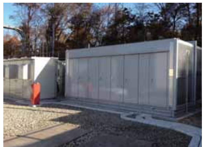
Regenerative energy storage system supplied to Haijima Substation of East Japan Railway Company's Ome Line [battery housing (left) and chopper (right)]
