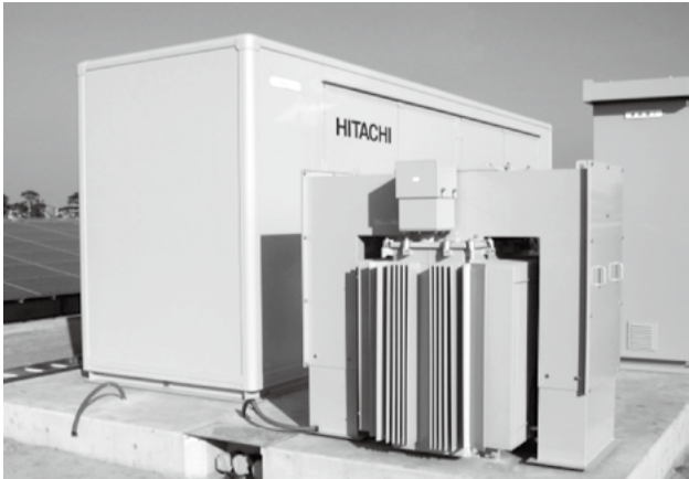
Fig. 7—Super Amorphous X ce Series Installation. Safety is improved by enclosing live parts inside a terminal box.
