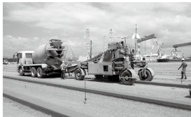
Fig. 8—Use of Slipforming to Lay Foundations.
