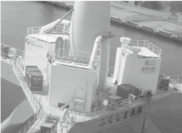
Fig. 9—Containers on Deck of Floater. The extra-high-voltage panel container is on the left, the high-voltage panel container is in the center, and the step-up transformer container is on the right (photograph courtesy of Fukushima Offshore Wind Consortium).
