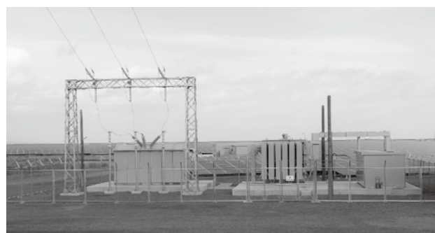
Fig. 3—Extra-high-tension Substation (Grid Connection Substation).
