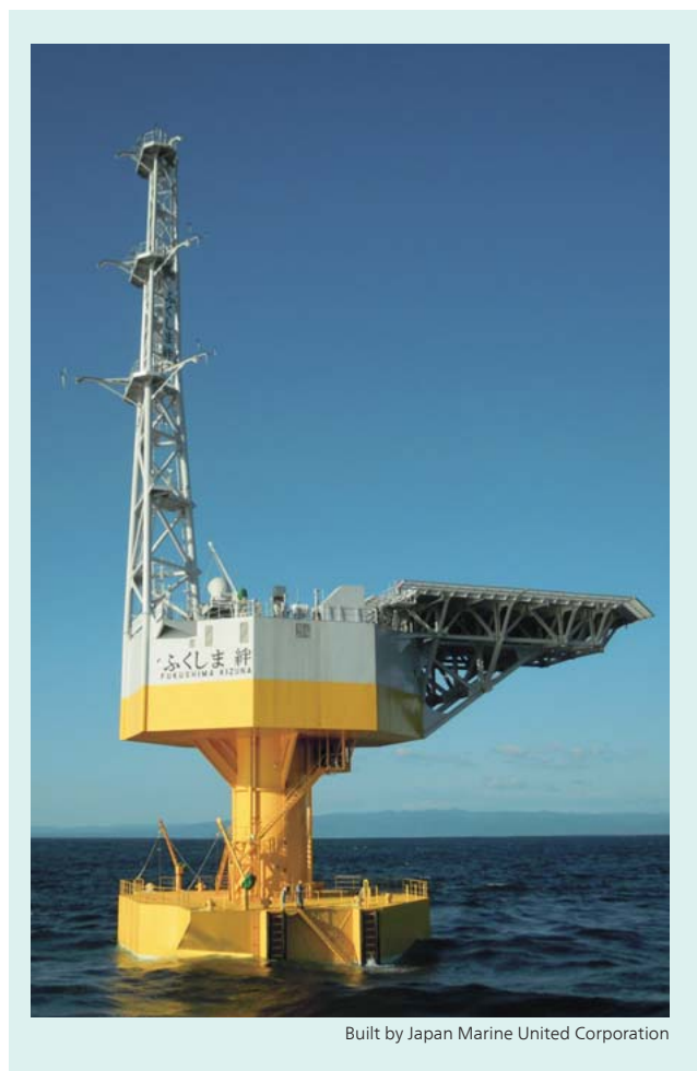
11 Floating offshore substation [The electrical conversion equipment is installed on the superstructure (painted white).]
