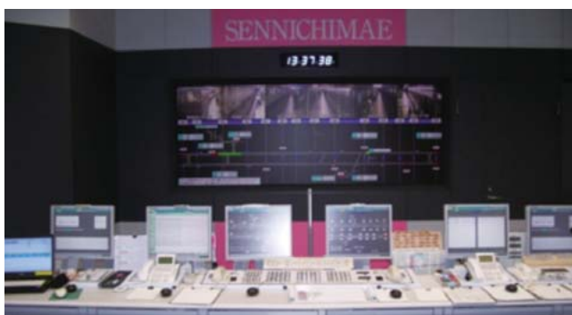
9 Traffic display panel and controller desk for Sennichimae Line
