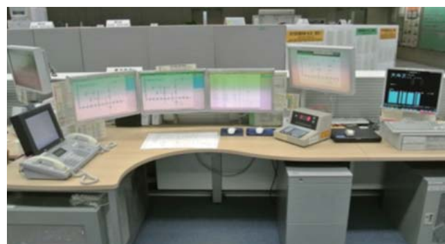
10 Control room and desk for new power supervision system
