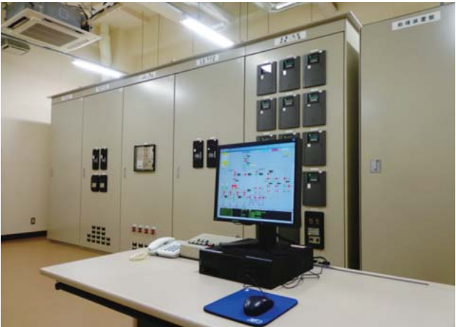
3 Portable substation (top), and power management system and protection interface panels (bottom)
