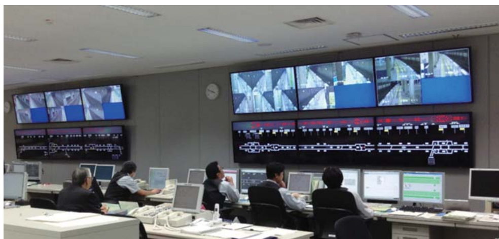
5 Traffic display panels and controller desks that form part of the traffic control systems for four Toei Subway Lines of the Bureau of Transportation, Tokyo Metropolitan Government
