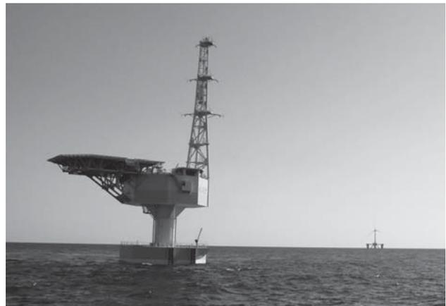
Fig. 9—Photograph of Exterior of Offshore Substation. The substation has one 66-kV incoming line and transformer output of 25 MVA. Its equipment is housed within the upper deck. This photograph was taken off the coast of Onahama, Fukushima Prefecture. The substation is shown in the foreground, with a 2-MW Hitachi wind turbine in the background (photo courtesy of the Fukushima Offshore Wind Consortium).
