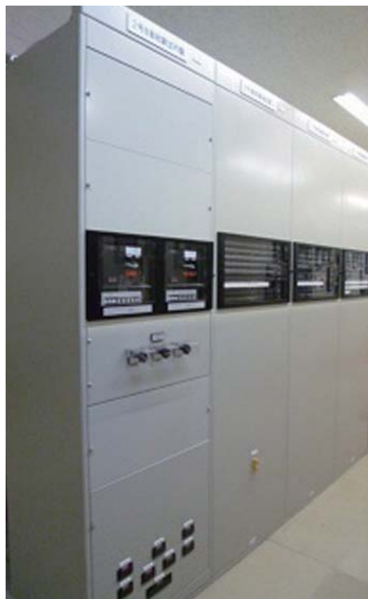
4 Upgraded protection relay panel
